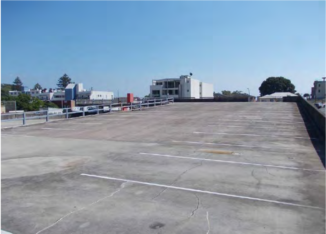
View of Top Deck of Car Park from Donald Street End
