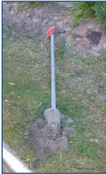
Traffic signs ripped out
