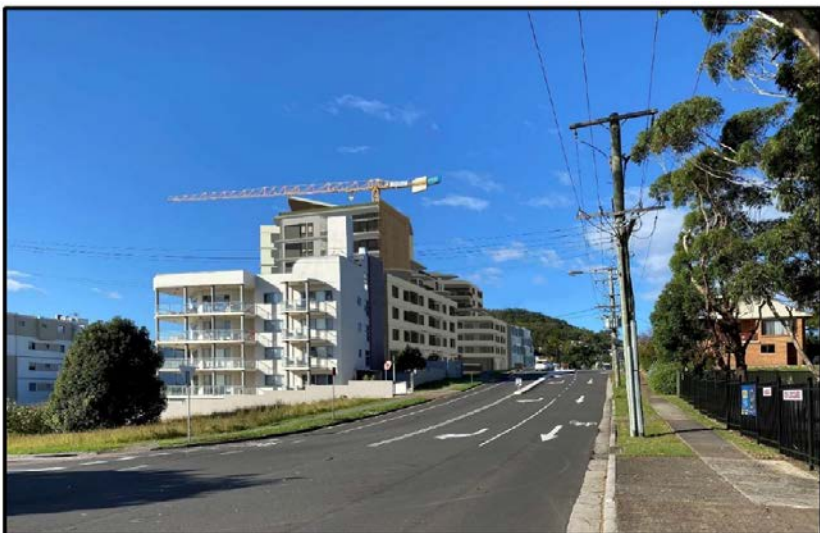
Image 5: Proposed development site (existing crane included).
