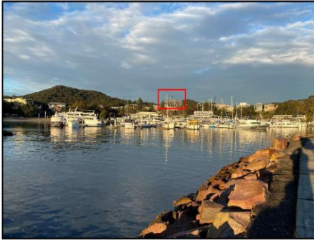
Image 1: View towards the site (existing crane included).
